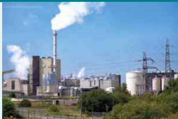
Shotton paper mill is saving CO 2 with a biomass Combined Heat and Power plant
