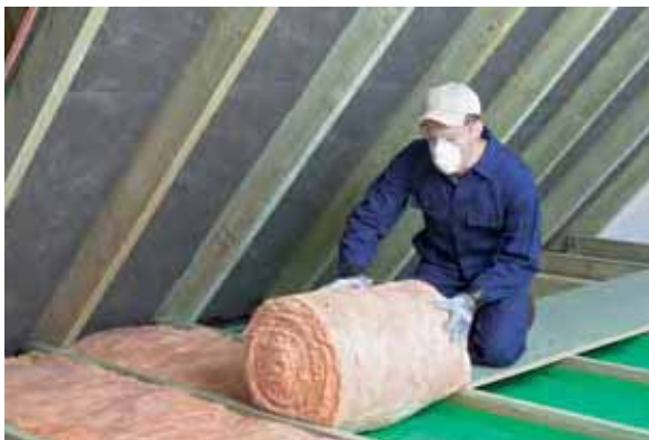
The Government is committed to helping six million households insulate their homes by the end of 2011
